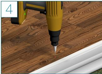
Remove the Base Rail and use a <sup>3</sup>/<sub>8</sub>" drill bit to drill 3<sup>1</sup>/<sub>2</sub>" down in each marked location
