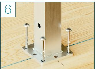
• Using the T-30 Torx Bit, screw the post mounting screws down snug through the post foot
