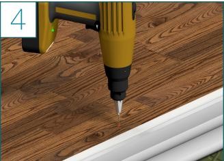
• Remove the base rail and use a 3/8" drill bit to drill 31/2" down in each marked location
