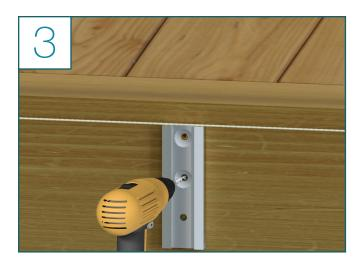
• Using a 1/4" drill bit, predrill all 3 holes
