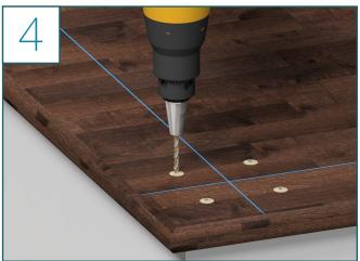
Use a <sup>3</sup>/<sub>16</sub>" drill bit to pre-drill the post mounting holes to an approximate depth of 3<sup>1</sup>/<sub>2</sub>"
