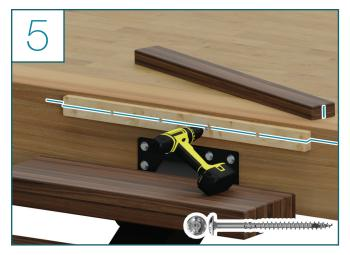
• Mount the nosing blocking using a single provided  $$^{5}\!/_{16}"$ x 6" RSS screw in one of the two center holes$
