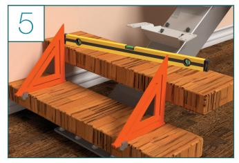
• Use a level to ensure the tread is plumb
