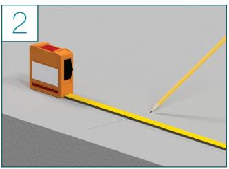
Using a pencil, mark the center of where you want each post to be positioned
