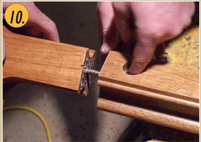
Hold plastic washer inside 1" hole from step 6. Insert machine end of RAIL BOLT into 5/16" hole from step 5.
