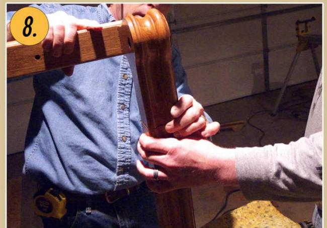
**8.** Without using any glue, insert machine end of RAIL BOLT into 5/16" hole from step 5 to make sure everything lines up properly.
