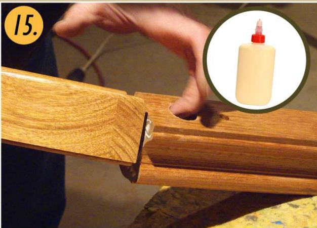
Assuming the parts from step 14 line up, partially unscrew the nut from the RAIL BOLT and apply wood glue between the handrail & fitting.
