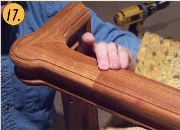
Minor sanding may be required for handrail and fitting to come together perfectly.
