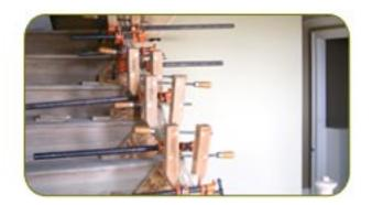
Allow the handrail to sit for 24-48 hours before removing the clamps. Plan to spend several hours with a chisel and sandpaper removing glue and shaping the handrail.
