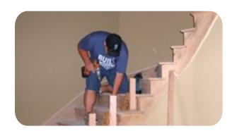
Construct angle brackets from any strong and straight construction material. The angle brackets will have a lot of force against them so take your time and make them very strong. The base that is screwed to the tread should be a minimum 3" wide and 12" long. The vertical should be a minimum 3" wide and 12" long.
