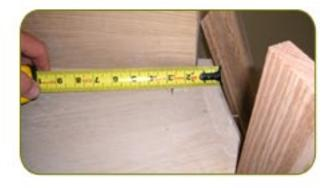
Layout the location for your handrail and install angle brackets with at least 4 screws into the stair treads. If the handrail is being bent while disposable construction treads are in place, be sure that the construction treads are firmly attached. If the angle brackets are attached directly to the final treads, then the holes in the stair treads can be filled and sanded after installation.
