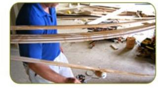
Wet the handrail with water and pre-bend it by placing it against the brackets and clamping it. Wet the bending mould as well so that it will become flexible. If the handrail is being installed around a tight radius then apply several applications of water to make the handrail more pliable. Bend the handrail gently by increasing the clamp pressure over a 48 hours.
