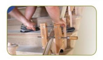
Put the handrail into place and check to make sure it is centered so that there is adequate overhang on each end. Place the first clamp in the center of the bend and begin working outward placing a clamp every other step.
