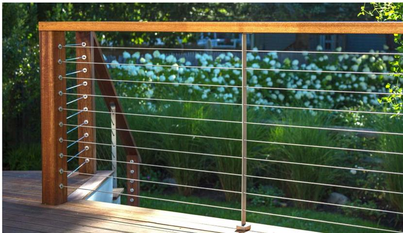
*The intermediate posts in the picture above are only used between wood posts*
